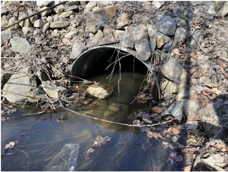
Photo 9. Ditch 1 flows through a culvert under South Main Street.
